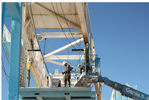
Installation of a rig, Wyoming
