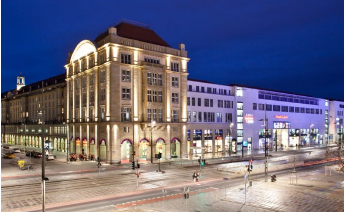
Altmarkt-Galerie, Dresden: A historic, listed building meets accessible shopping center architecture.
