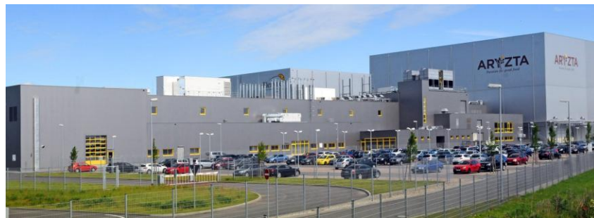
ARYZTA manufacturing facility in Eisleben, Germany
