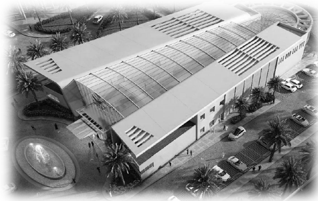
Kuwait: Ahmadi Innovation Valley Center (AIV) Under Construction (Estimated 2026)
