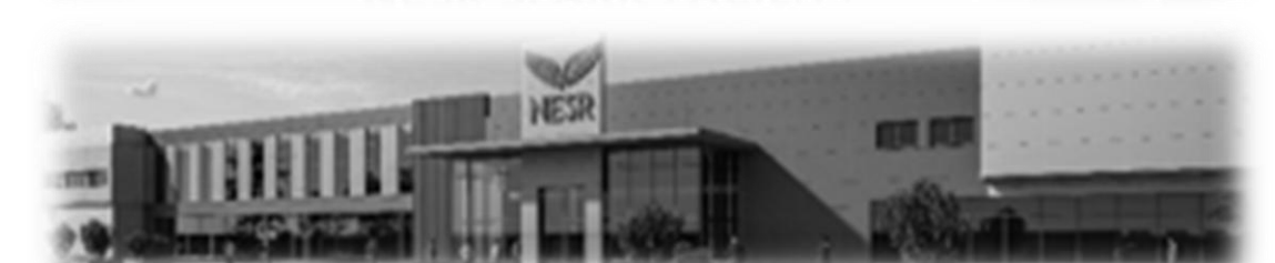
Saudi Arabia: King Salman Energy Park Ops Facility (SPARK) Under Construction (Estimated 2026 to support Jafurah Ops)
