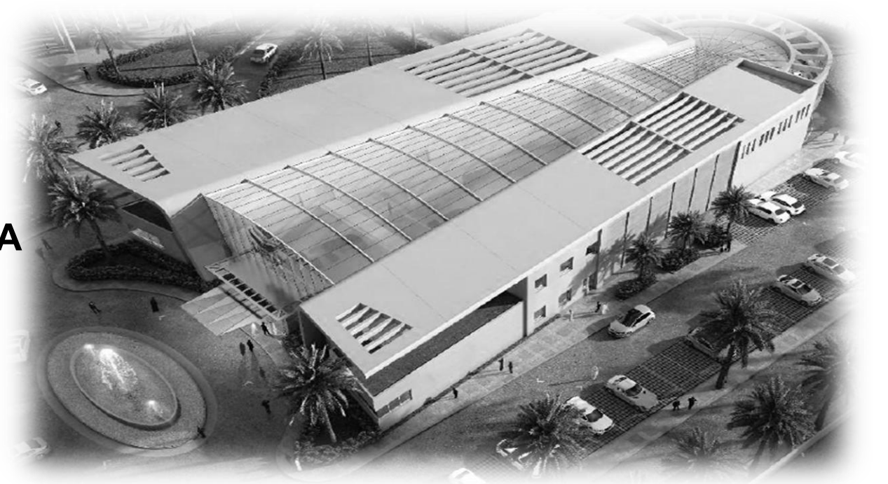
Kuwait: Ahmadi Innovation Valley Center (AIV) Under Construction (Estimated 2026)
