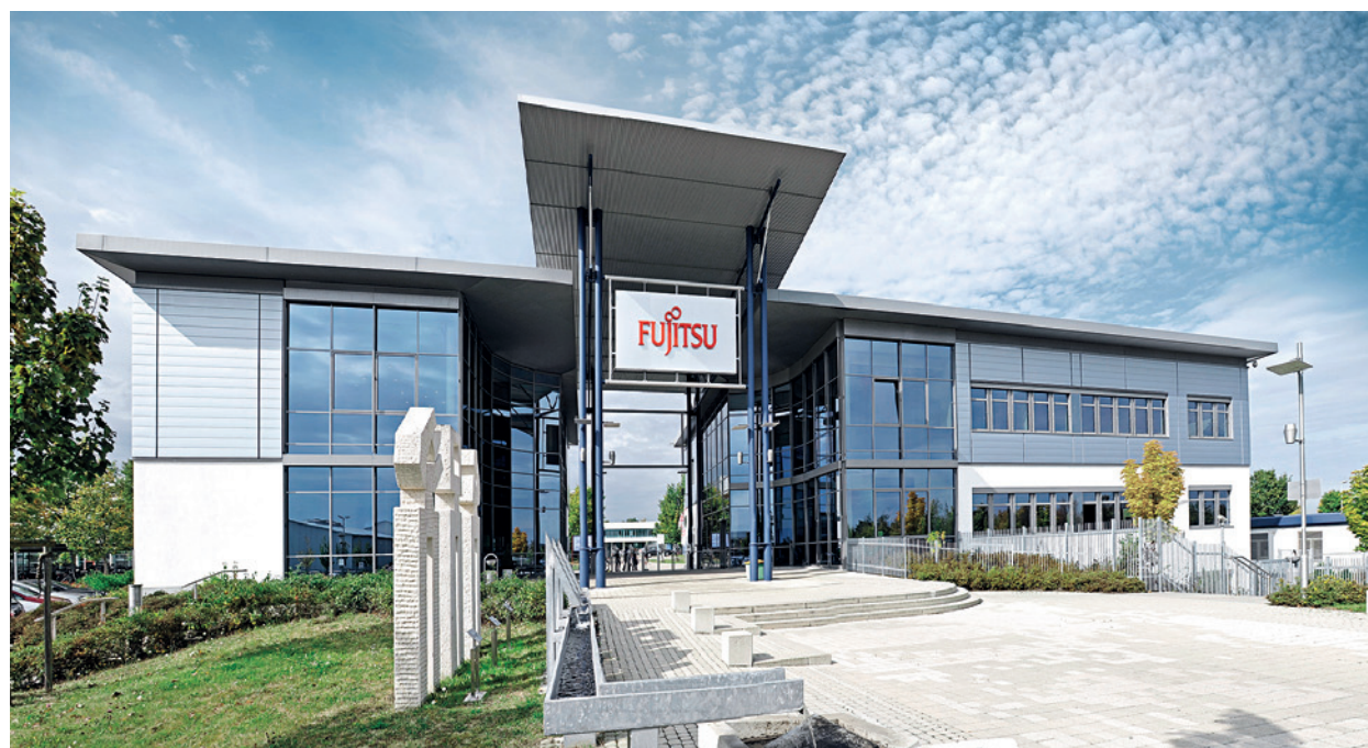
Fujitsu Technology Solutions GmbH Werk Augsburg
