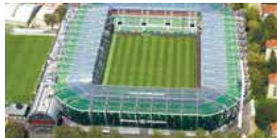
PRECAST Allianz Stadium, Austria
