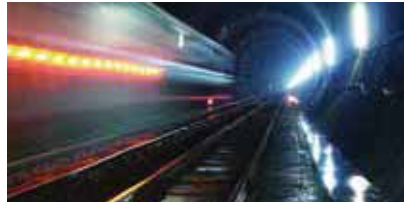
ALLPLAN Gotthard Base Tunnel, Switzerland
