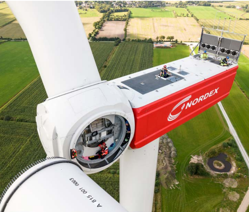
The N163/5.X turbine is installed at the Janneby citizen wind farm in Germany.
