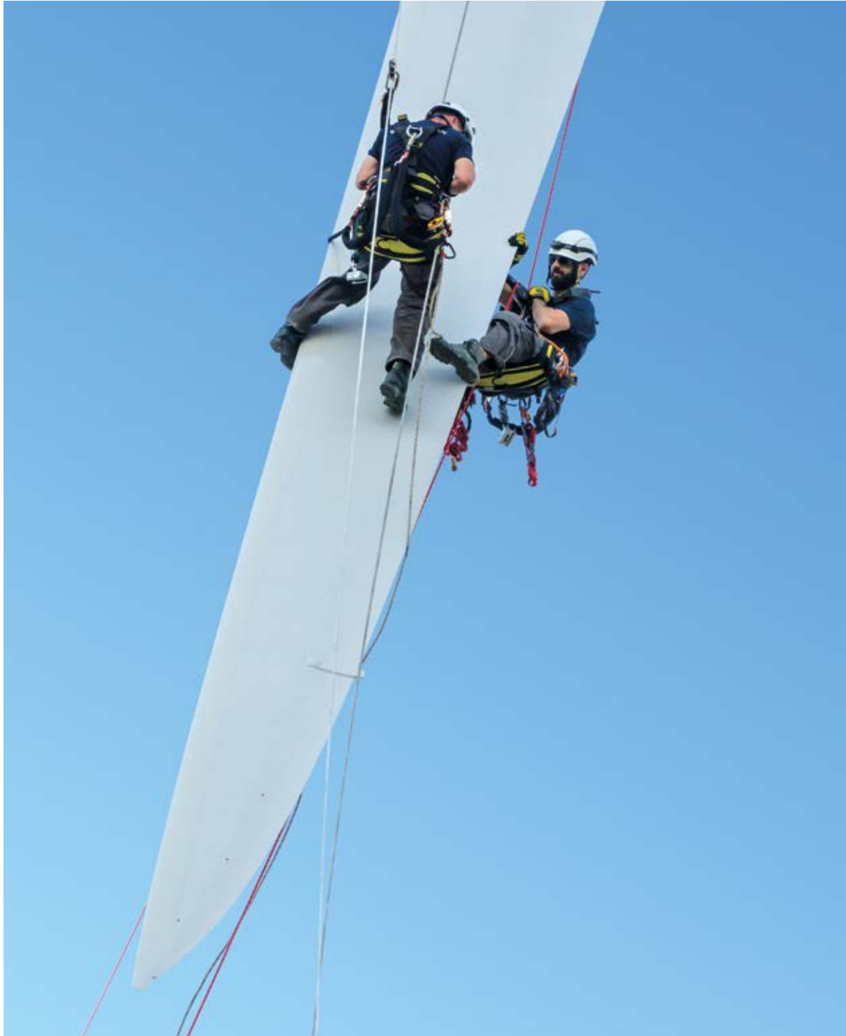
Safety First! Service technicians inspecting rotor blades
