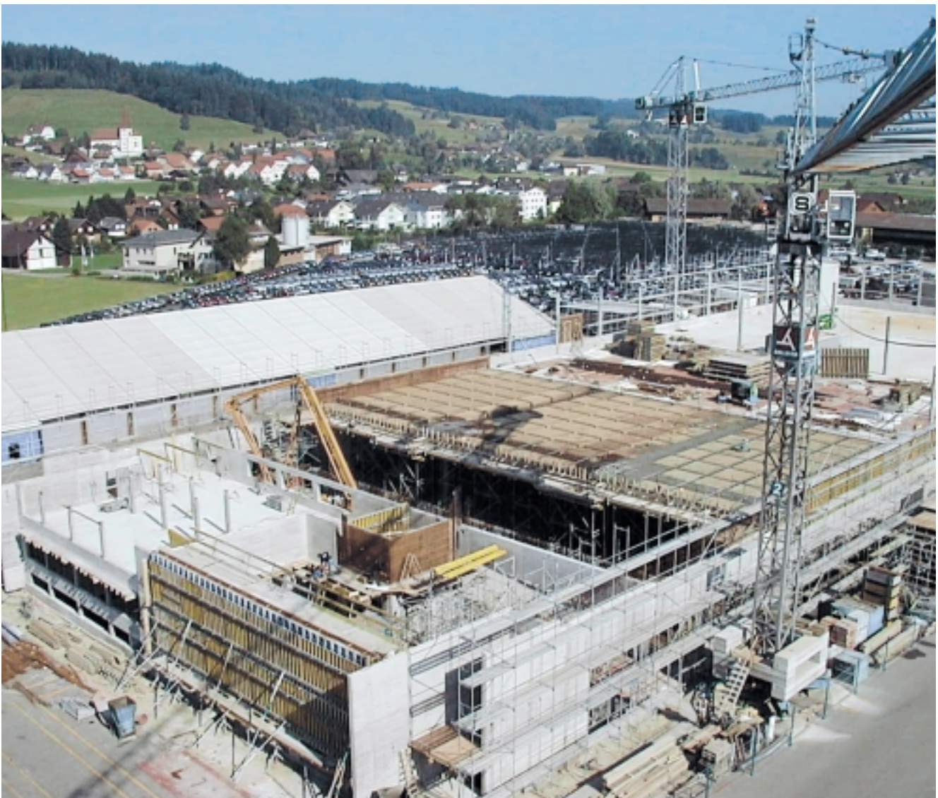
Construction site of our customer Anliker AG in Altishofen, Switzerland
