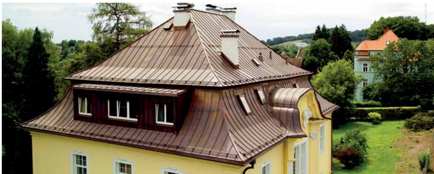
Renovated rooftop of a mansion in Linz (copper strip)
