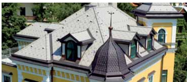
Renovated rooftop of a mansion in the Salzkammergut, Austria (eternit shingles and copper)
