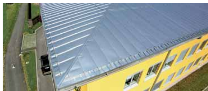
New building of a technology centre in the Salzkammergut, Austria (aluminium coated strip)
