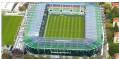
PRECAST Allianz Stadium, Austria
