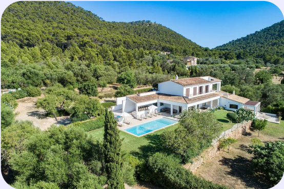
House in Port d'Andratx (Mallorca, Spain)
