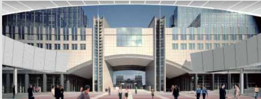
SCIA.ESA PT - used to design the new footbridge at the European Parliament
