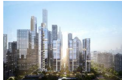
Super Headquarters Base project, Shenzhen
