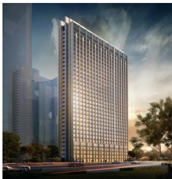
Zhengzhou Huiji District Project
