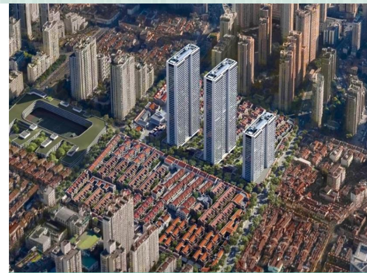
Shanghai·East Jianguo Road urban renewal project
