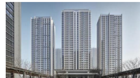
Qingdao Taixing Road Project
