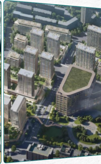
Haichao Road Project, Hangzhou
