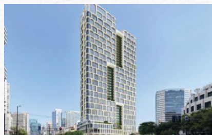
East Siminli project, Shanghai
