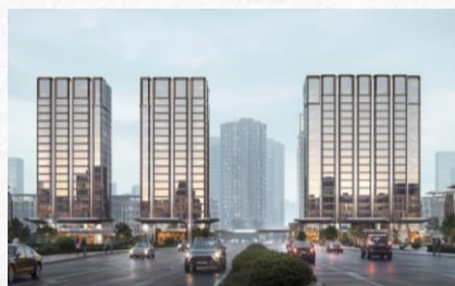
Haichao Road TOD project, Hangzhou
