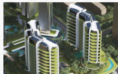
Super Headquarters Base East project, Shenzhen
