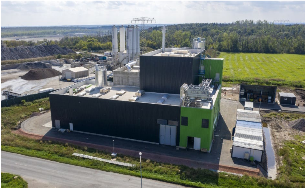
Thermal sludge treatment plant in Halle-Lochau (Germany)
