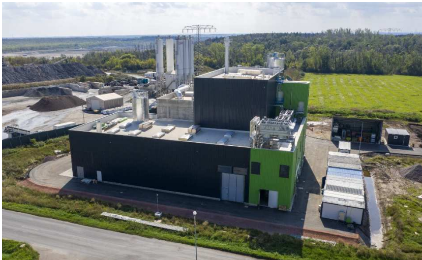
Thermal sludge treatment plant in Halle-Lochau (Germany)
