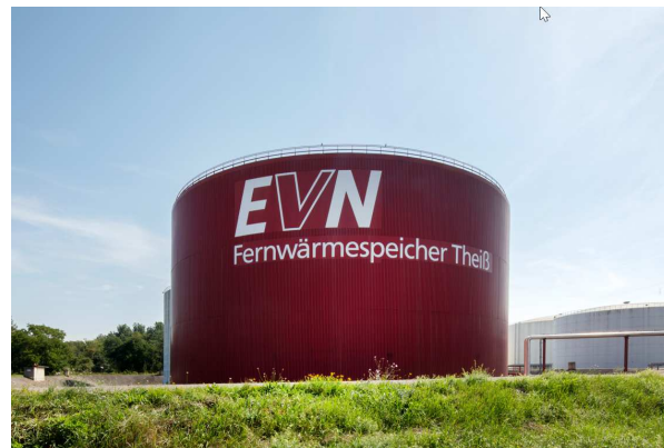
Hot water storage
