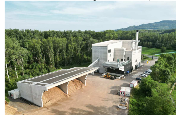
Biomass-fired cogeneration plant
