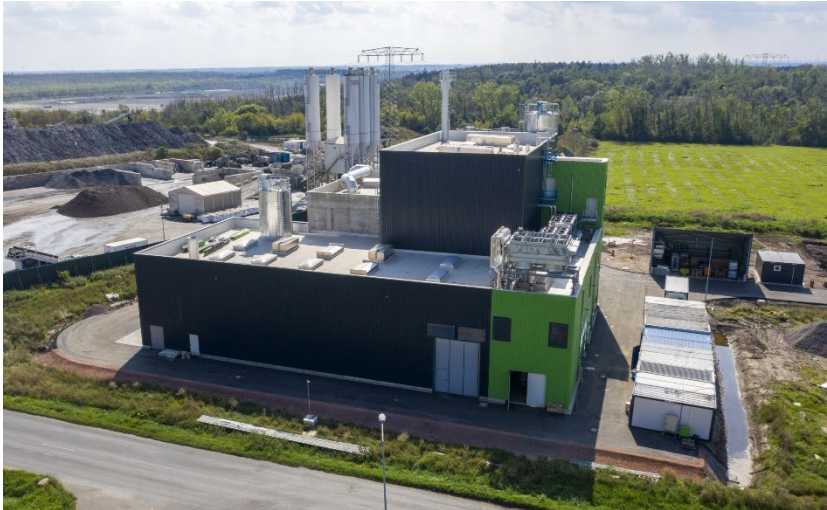
Thermal sludge treatment plant in Halle-Lochau (Germany)
